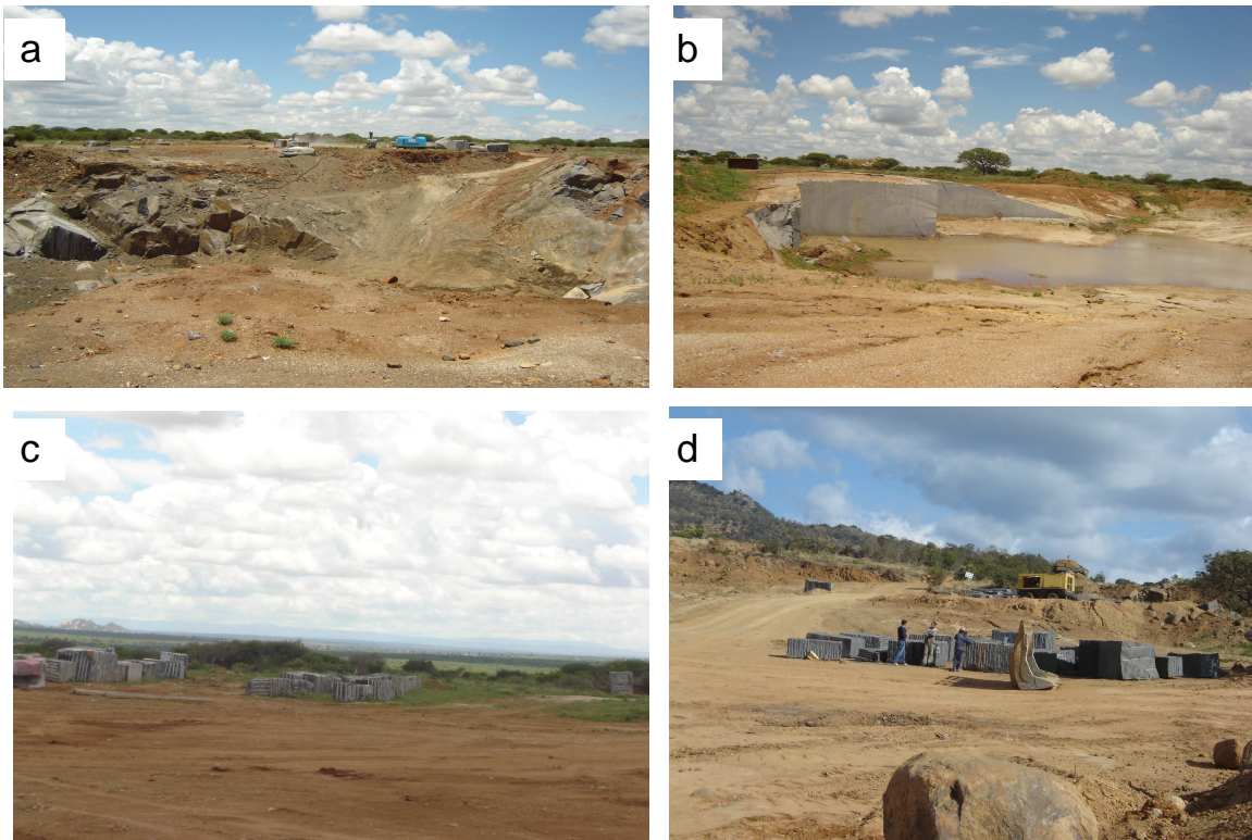
Fig. 8. Granite workings at the Earthstone Granite and Phalaborwene Marble and Granite. Site preparation to open up the granite; (b) granite face ready for granite block extraction (c) Granite blocks ready for processing or for transportation to a processing plant or selling (d) Black granite blocks from Phalaborwene Marble and Granite.
